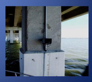
6. Electrochemical Chloride Extraction (ECE)
